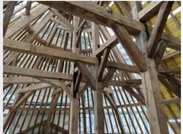
Company Asselin : Chantier Vannes
